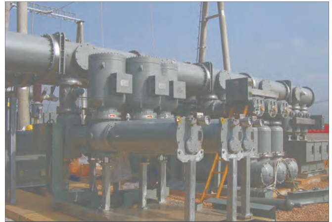
252kV Gas Insulated Switchgear
