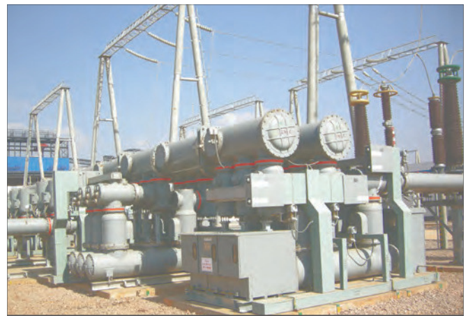
252kV Gas Insulated Switchgear
