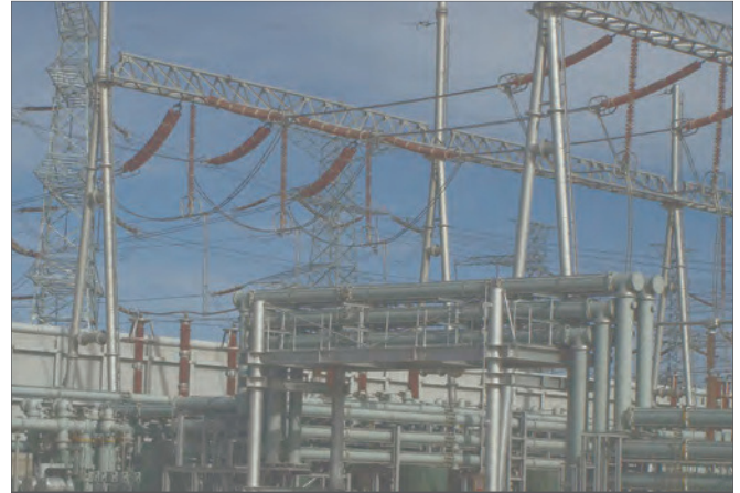
363kV Gas Insulated Switchgear at Golmud Substation
