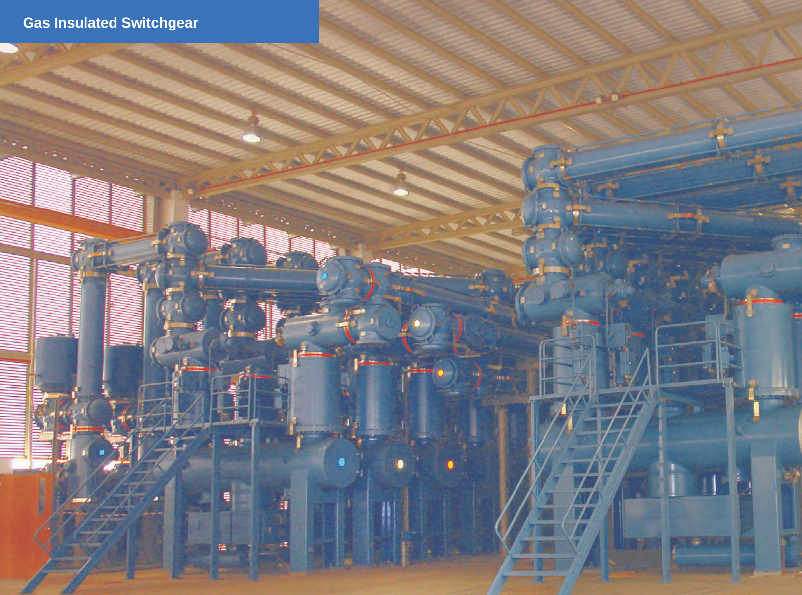
420kV Gas Insulated Switchgear
