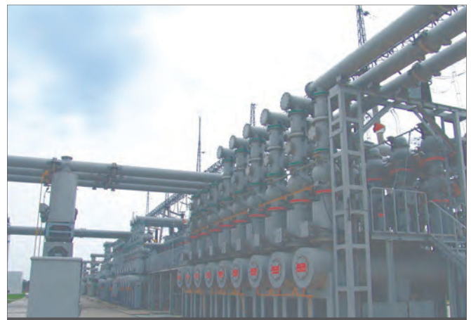
363kV Gas Insulated Switchgear in Weenan, Shaanxi
