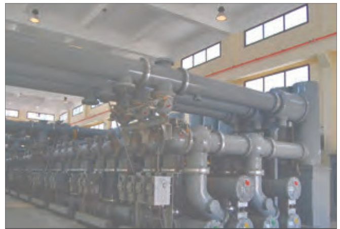
363kV Gas Insulated Switchgear
