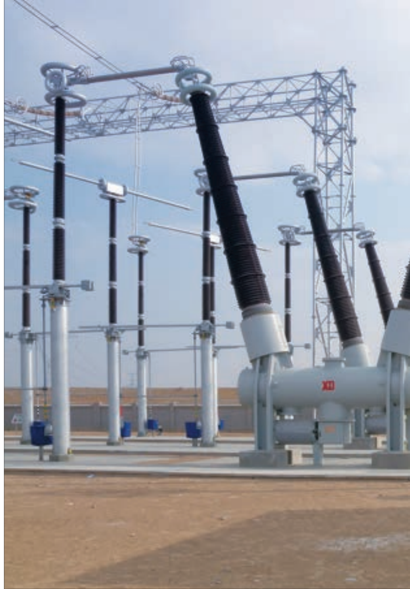
800kV Dead Tank SF 6 Circuit Breaker
