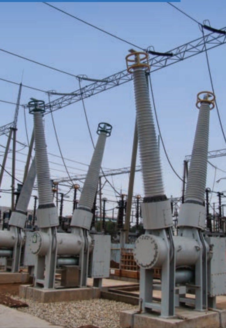
363kV Dead Tank SF 6 Circuit Breaker
