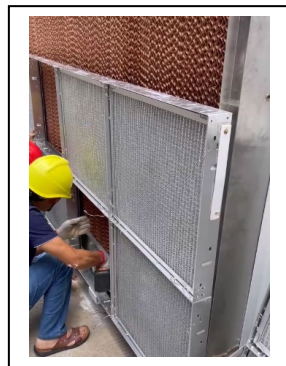
Air Filters Installation
